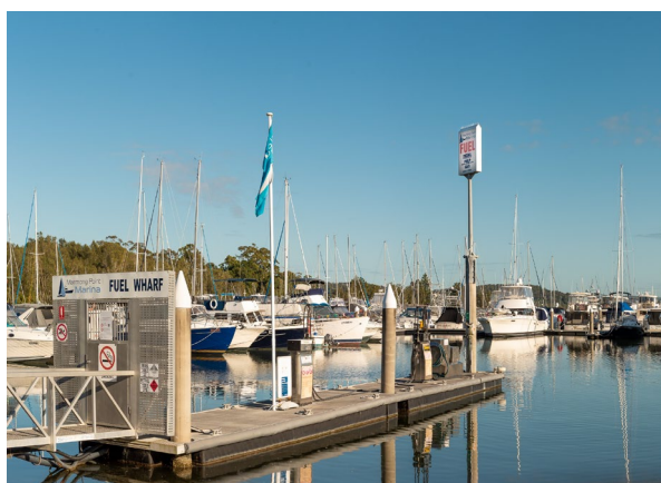
Vessel pumpout and fuel wharf
